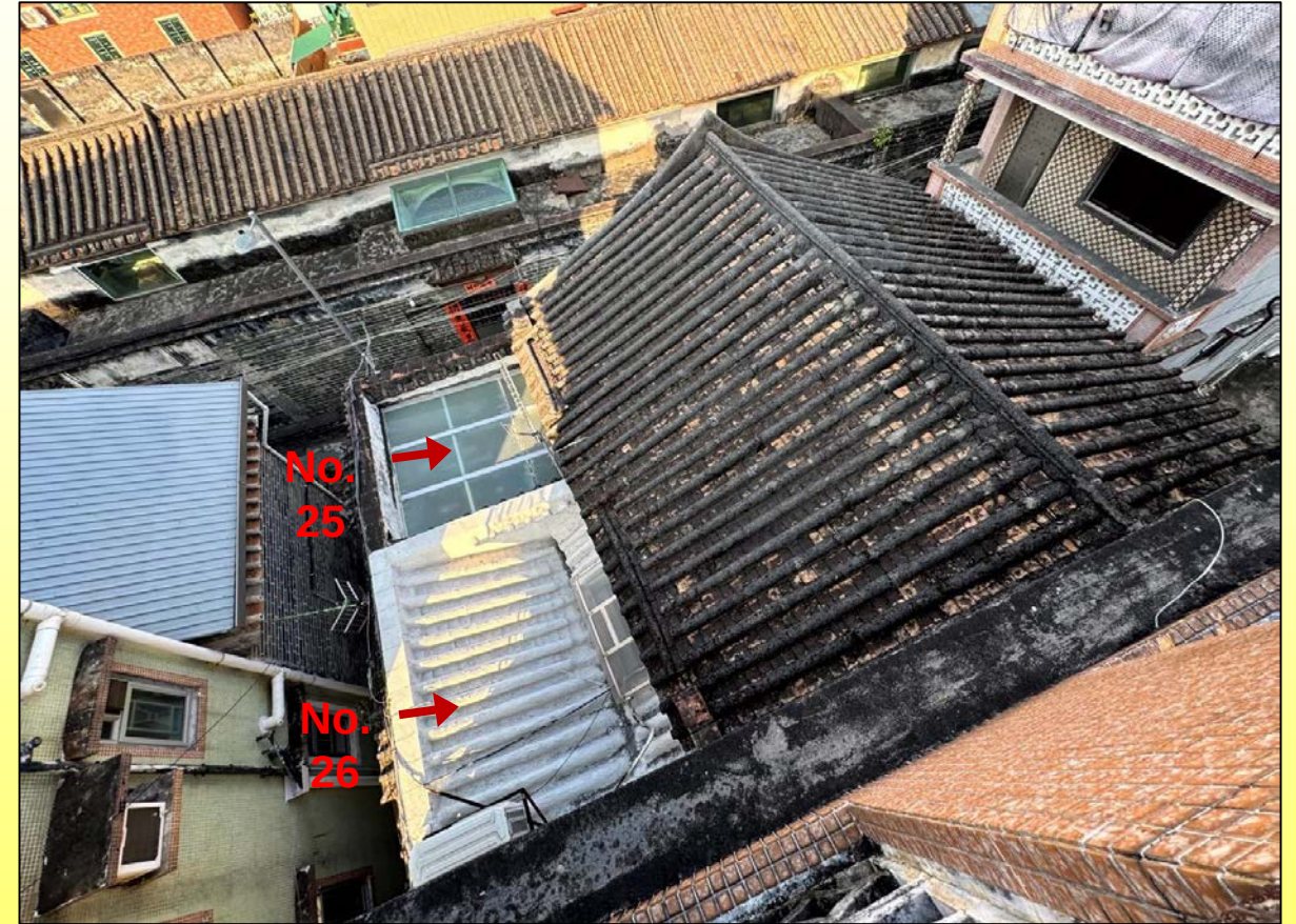
村屋的屋頂 Roof of the Houses
